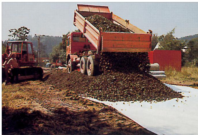
△ **HaTe®**-nonwovens used in separation reduce the need for subbase, increase the bearing capacity of the subgrade and can be installed without difficulty.
