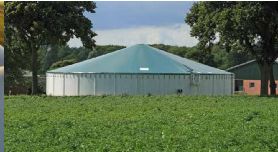
Weatherproof silo cover on element tank, Uedem in Germany
