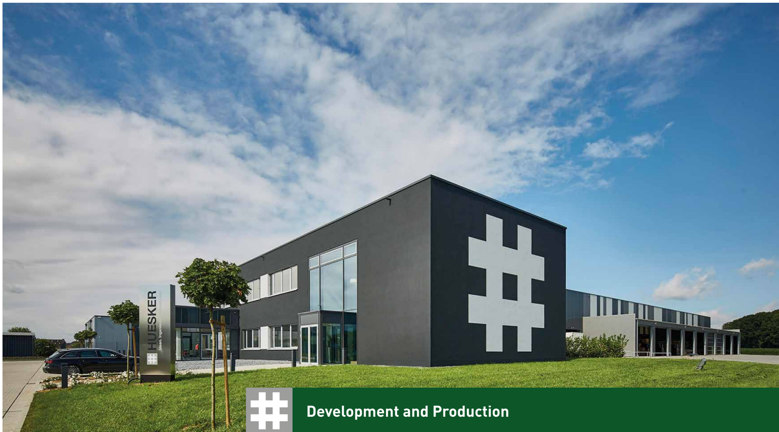
Exterior view of the office building in Duellen
