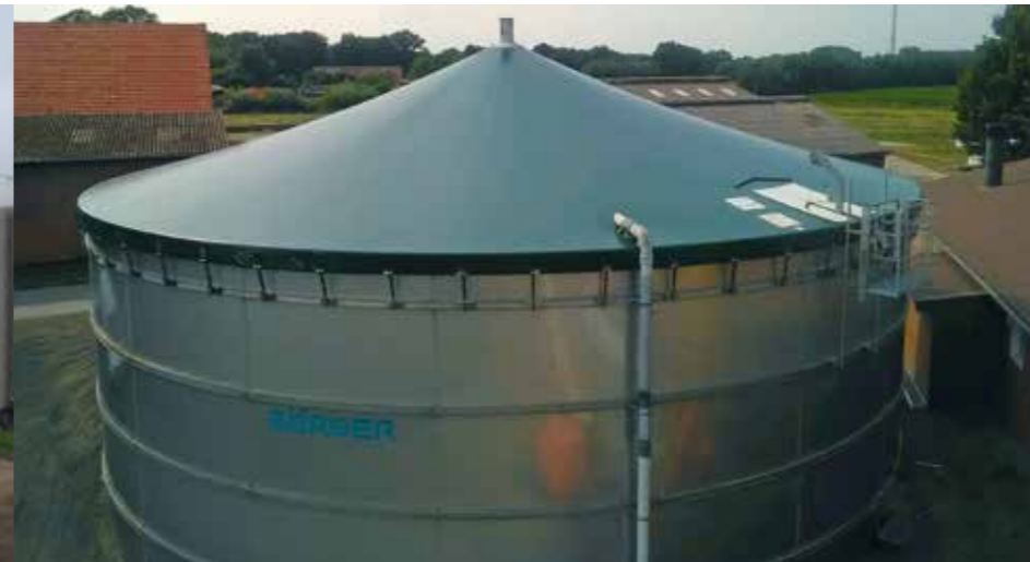
Weatherproof silo cover on steel tank, Heek in Germany
