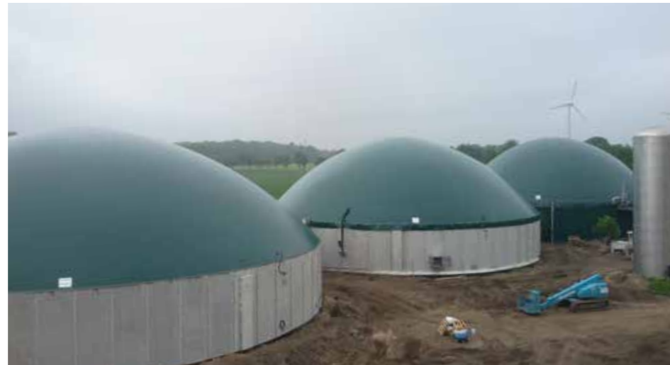
Double membrane roofs on element tank, Cappel in Germany
