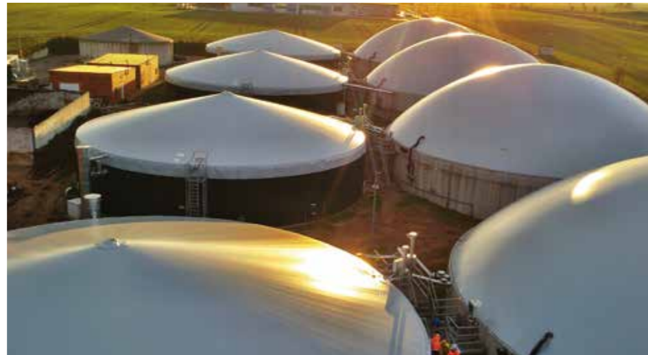
Double membrane roofs & silo covers single-skin gas tight on element tanks, Koennern in Germany
