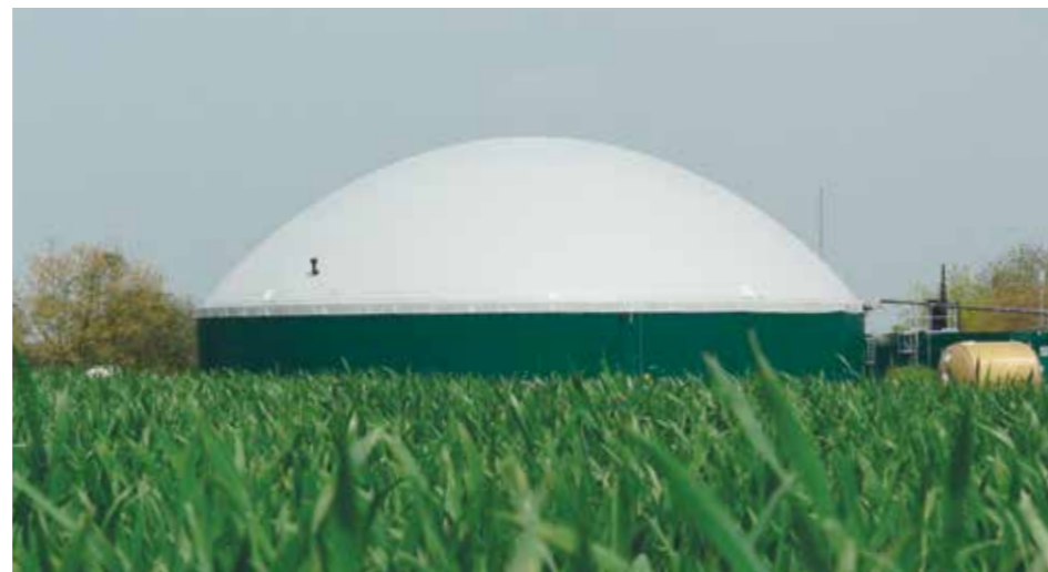
Double membrane roof on concrete tank, Grefrath in Germany
