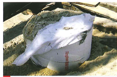
Figure 6 Recently installed sand-filled geotextile-encased column (GEC) using Ringtrac® 100/250.
