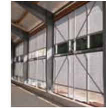
Lubratec Double Roll-Up Ventilation bottom opening
