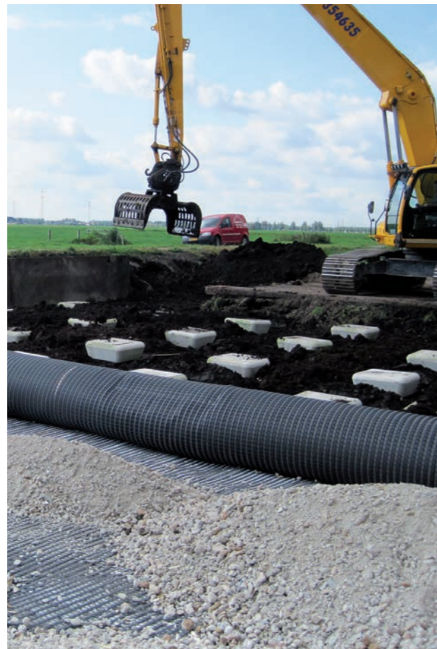
Geotextile reinforcement installed on piles (N 210; Netherlands)
