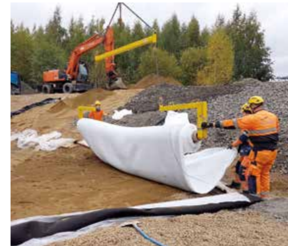
Precipitation treatment Finland | Precipitation runoff from sealed surfaces contaminated with PAHs and CHCs is treated in a stormwater retention basin. By installing Tektoseal Active AS and AC in the bottom of the pool, pollutants are filtered out of the water before it seeps away. The basin walls are largely impermeable to water and lined with a clay liner.
