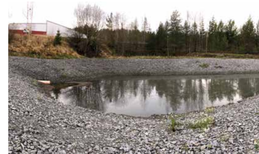
Mine water treatment in mining Finland | Water containing metal can also be treated in basins in the mining industry. For mine water treatment in a closed nickel mine, two filter basins were lined with Tektoseal Active HM.
