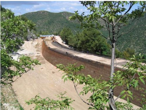
Figure 7. Trapezoidal embankment during construction (basin side inclined 80°)
