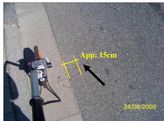
Figure 3. Lateral crack at the edge
