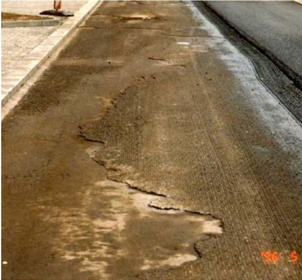
Figure 2. Surface after milling
