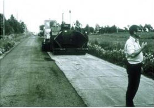
Figure 1. One of the first attempts to use a geogrid in asphalt pavement at the early 1970s
