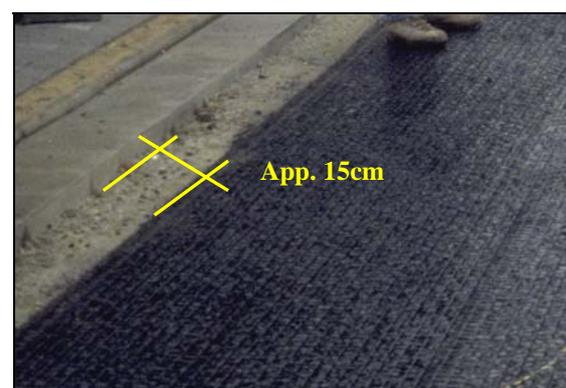
Figure 4. Fitted reinforcement (detail)
