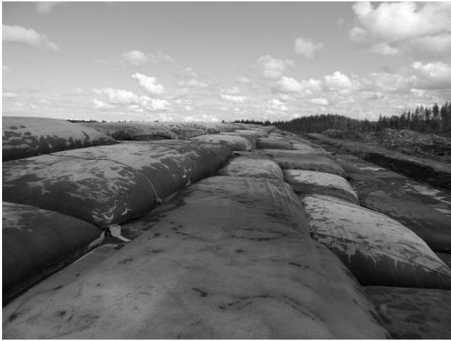
Figure 1. Stacked dewatered geotextile tubes (5 tube layers high) after Wilke et al 2015.
