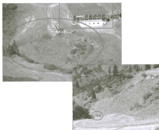
Figure 8. August 2014: left up: overview, reinforced slope is marked; right down: persons as a scale for the structure.
